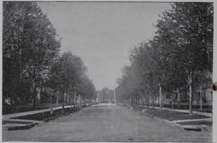
No. 2, CANFIELD AVENUE—West.
